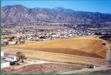
Construction of landfill underway.
