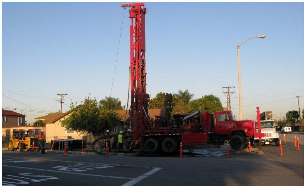
*Photo of drill rig conducting installation of water quality monitoring well at East Florence Place and Scout Avenue.*
