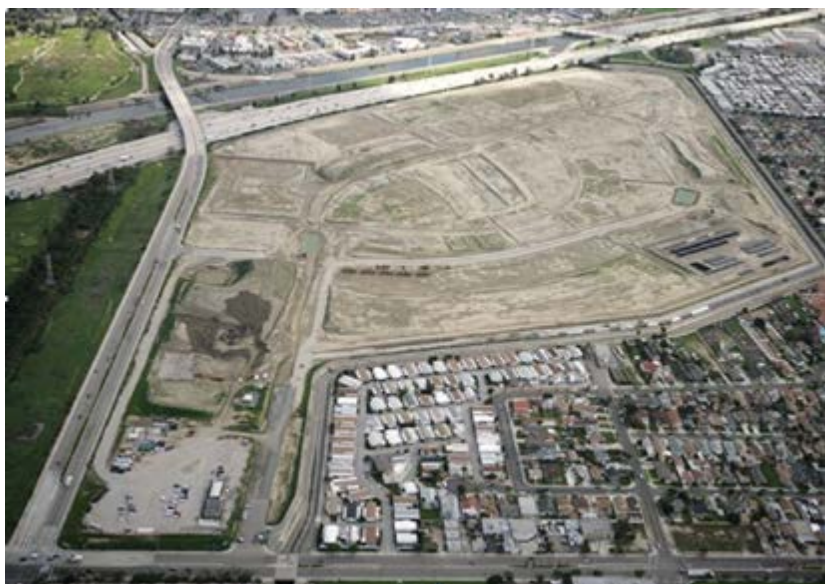
The former Cal Compact Landfill looking east towards Highway 405.
