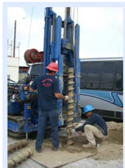
Workers prepare a monitoring well installation that will reach a depth of 130 feet.
