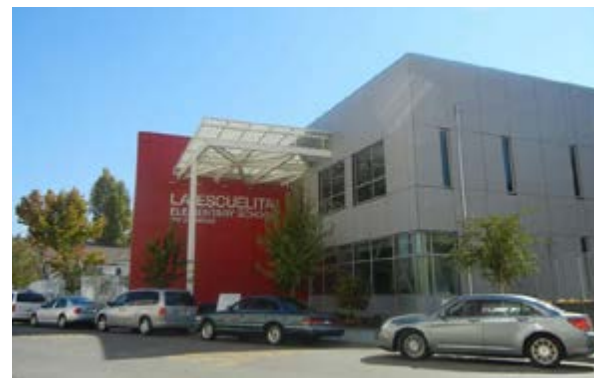
Top: Field work during Phase II of the La Escuelita Education Center cleanup in Oakland. Buildings in background is new construction completed after Phase I.
