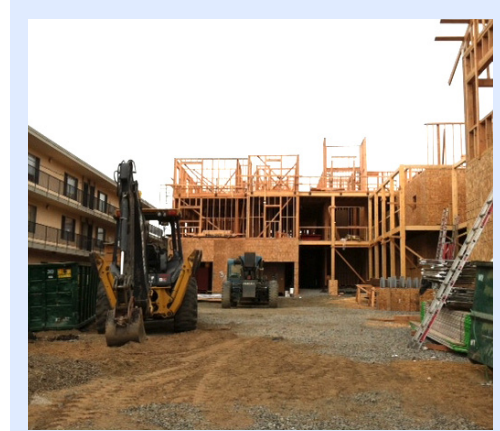
The complex under construction in Alameda.
