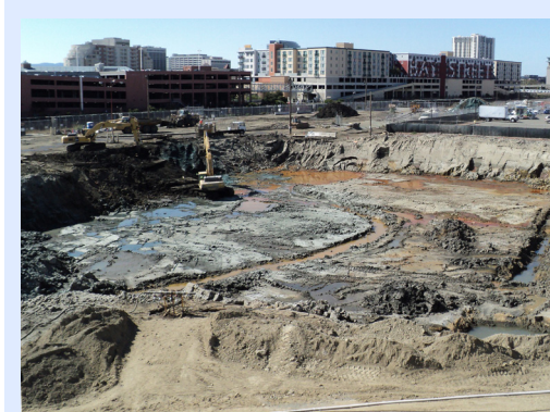
Excavation of the contaminated area.
